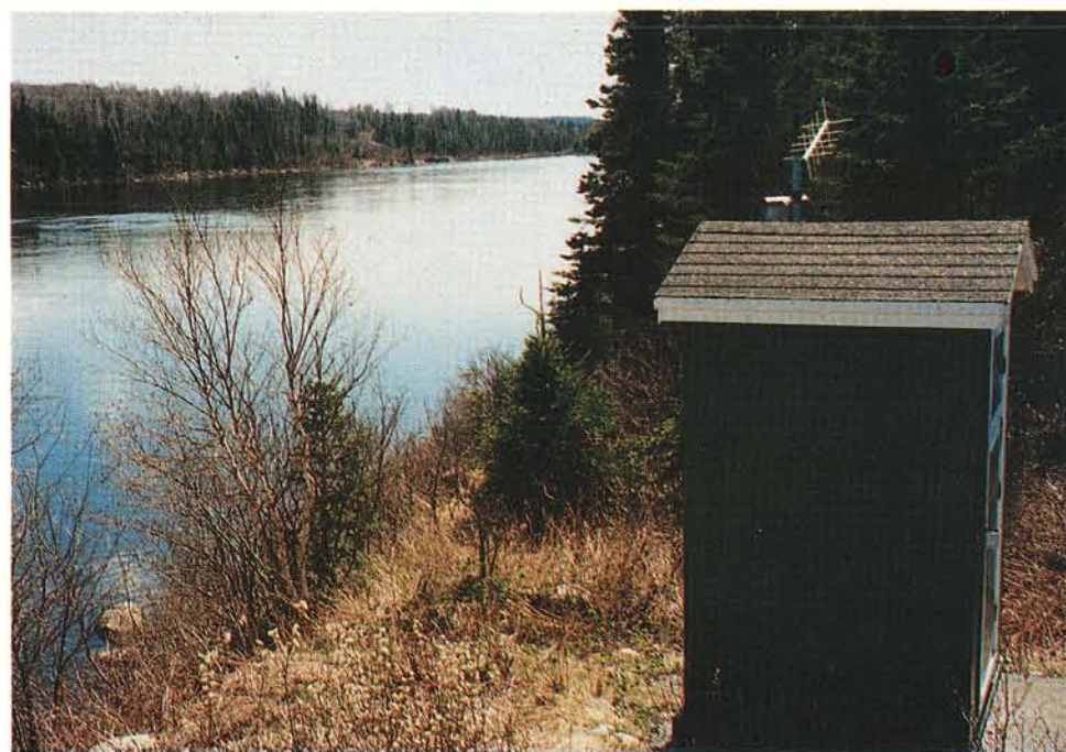
Figure 11.1 A Gauging Station with a Data Collection Platform. Note the antenna for data transmission via satellite.
