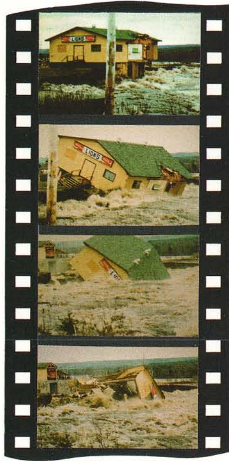
Figure 19.1 Heavy rain and snowmelt flooding in Bishop's Falls in 1983 resulted in severe damage.
